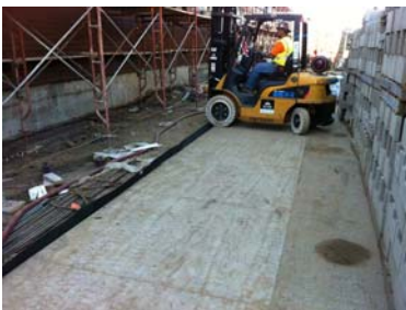
ProWattle at edge of sidewalk
