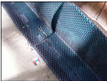
Anchored here with Masonry Nails
