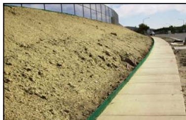
Protection at top and base of slope
