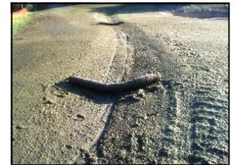
Fiber Rolls were installed first on the site and failed in the first storm
