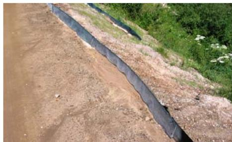
ERTEC spreads flow & captures sediment. It
