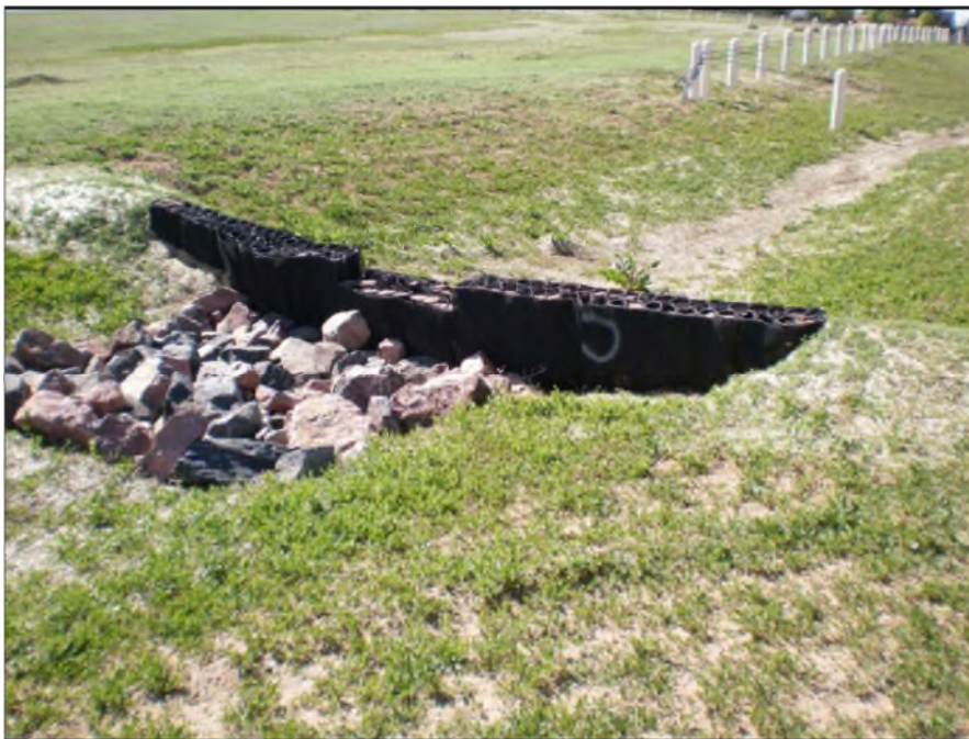
Figure 12: Finished Installation – Buckley Airforce Base – Colorado
