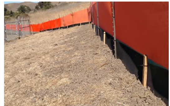
Sediment Control Installed to Control Run-On
