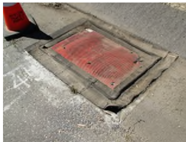
Year 2: Post storm—after cleaning. Grates do not need to be removed for installation or cleaning.
