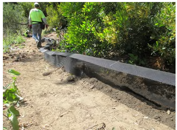
Photo 4: E-Fence™ with climber barrier
