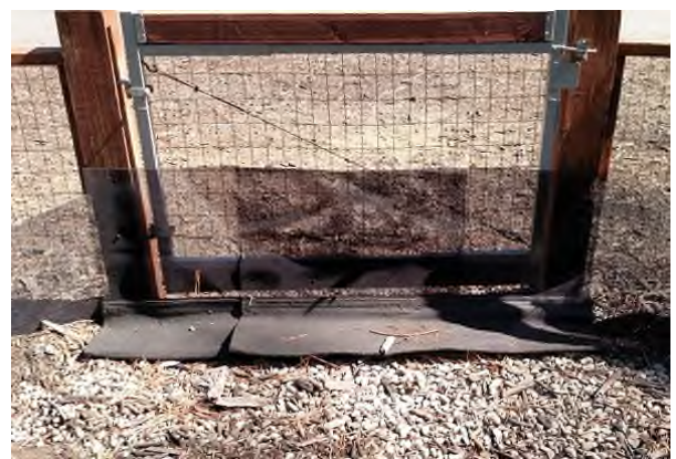
Photo 5: E-Fence™ gate panel with ground sweep for access gates
