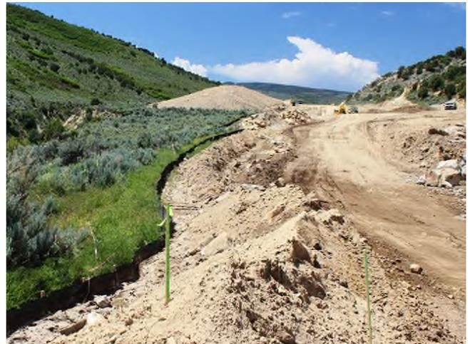
Collum Haul Road—S-Fence 20 installed along road
