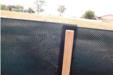
S-Fence™ is made from a heavy HDPE polymer matrix outer jacket and a specialized HDPE filter designed specifically for sediment control.
