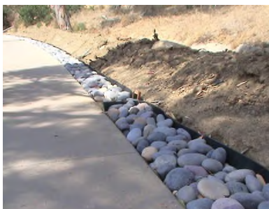
Edge Guard with rock, used as an effective edge treatment
