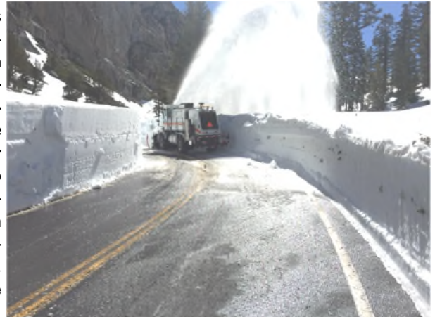
42,000 Linear Feet of ProWattle (8 miles) was installed in August, and by November it was buried, up to 10 feet in some areas, after record snow.
