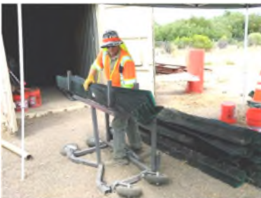
Installing Contractor removed ProWattle from this project and repackaged for reuse
