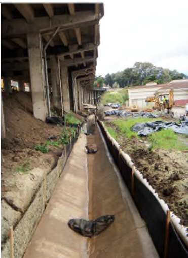
S-Fence installed on both sides of V-Ditch
