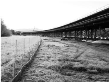
In many places, S-Fence was installed on existing silt fence posts after silt fence was destroyed.
