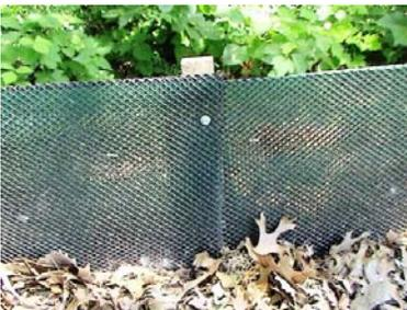
S-Fence is a 3 layer system. A rugged outer jacket houses a specialized sediment filter. 7' segments are overlapped and joint with wood stakes and nails. Wind driven knockovers are eliminated. Structural maintenance is eliminated. Maintenance is reduced to periodic removal of sediment to prepare for subsequent storms.
