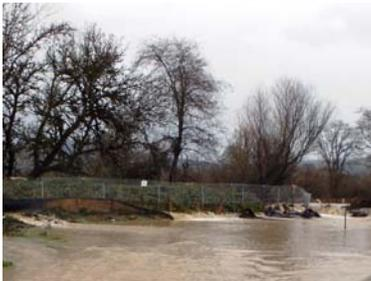
Thousands of feet of standard silt fence (above) was destroyed and replaced by S-Fence (below).
