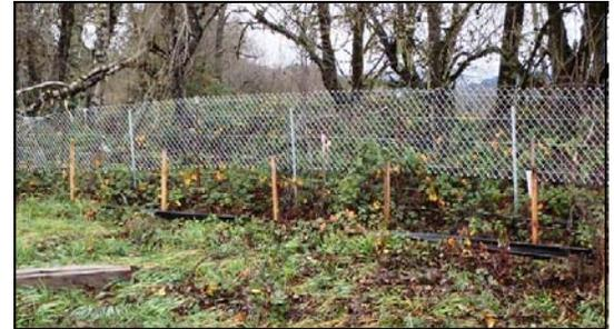
Over 11,000 LF of the original silt fence (initially installed by Caltrans) was destroyed during the storm of Dec 11, 2014.
