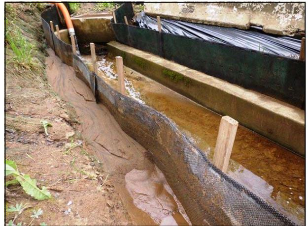
Particle filter allows water flow-through, and retains soil particles
