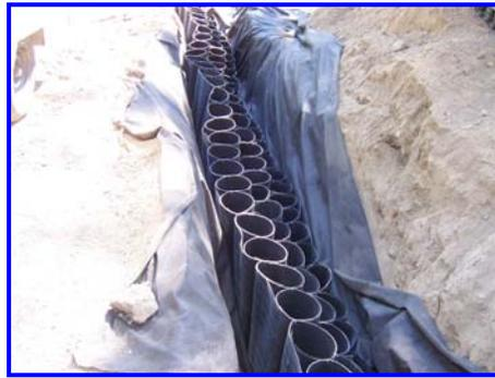
Figure 4: Section placement—post trenching—bank protection
