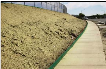
Protection at top and base of slope
