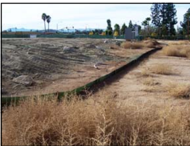
Perimeter & stockpile protection
