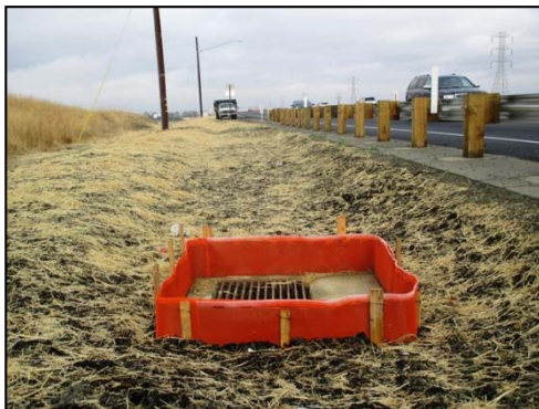
Road Construction – Roadside Ditch
