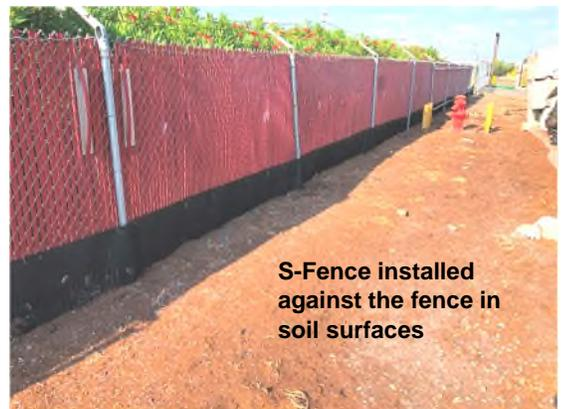
S-Fence installed against the fence in soil surfaces
