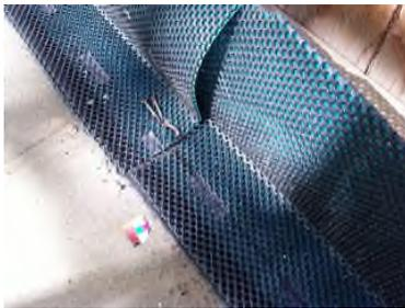
Anchored here with Masonry Nails
