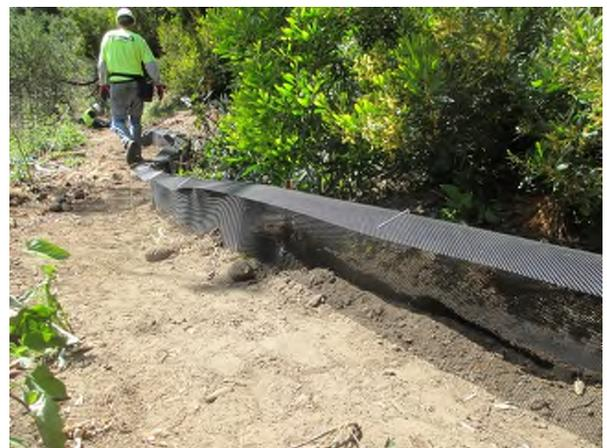
Photo 4: E-Fence™ with climber barrier
