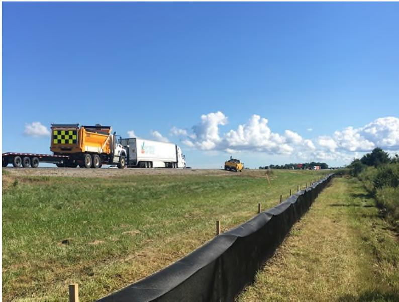
**E-Fence installed along the highway right-of-way to keep species at risk out of the construction zone**
