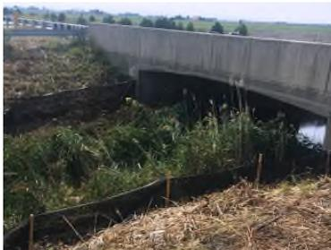
E-Fence shown connecting to and sealing against bridge abutments
