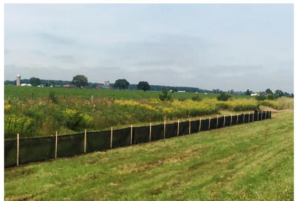
**E-Fence installed along the highway right-of-way to keep species at risk out of the construction zone**
