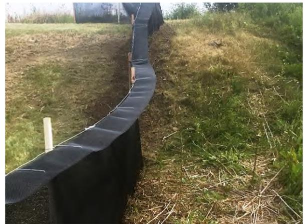
**E-Fence installed with an 8" climber barrier. The Eastern foxsnake is an excellent climber. It has been demonstrated that this species cannot climb E-Fence.**
