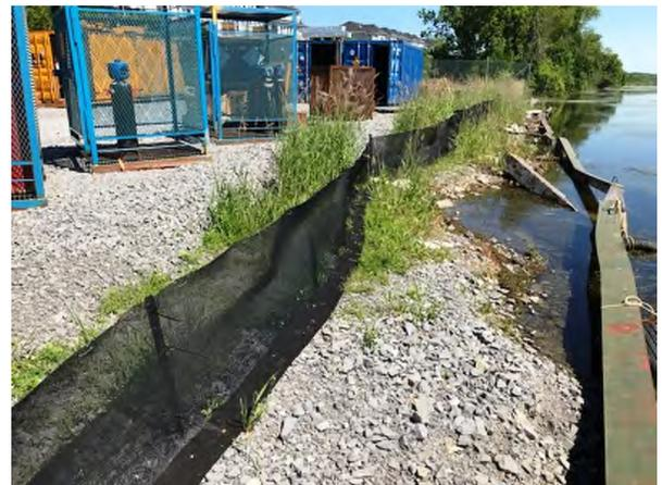
E-Fence installed with E-Fence No-Trench Ground Seal™ where trenching is difficult or unwanted
