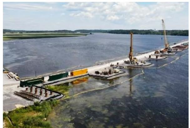
E-Fence installed along the fingers of the causeway to keep turtles out of the construction zone
